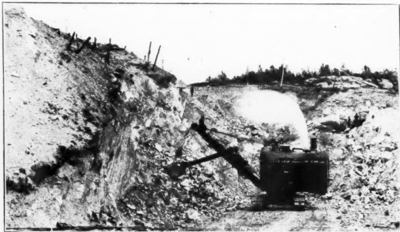
Shovel at Work in Pit, Showing Formation
